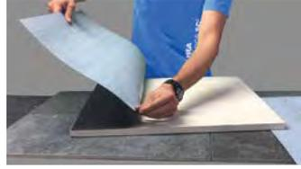
**2** Starting from one side, peel the protective foil, ensuring perfect adhesion of SHOCK CONTROL® to porcelain's surface.
