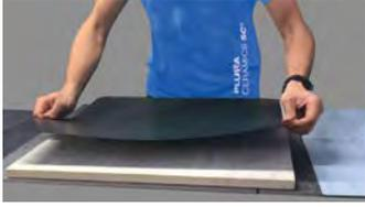
**1** Choose the proper size of SHOCK CONTROL® considering the size of the tile and apply it on the tile's lower surface, avoiding folds and aligning the edges.
